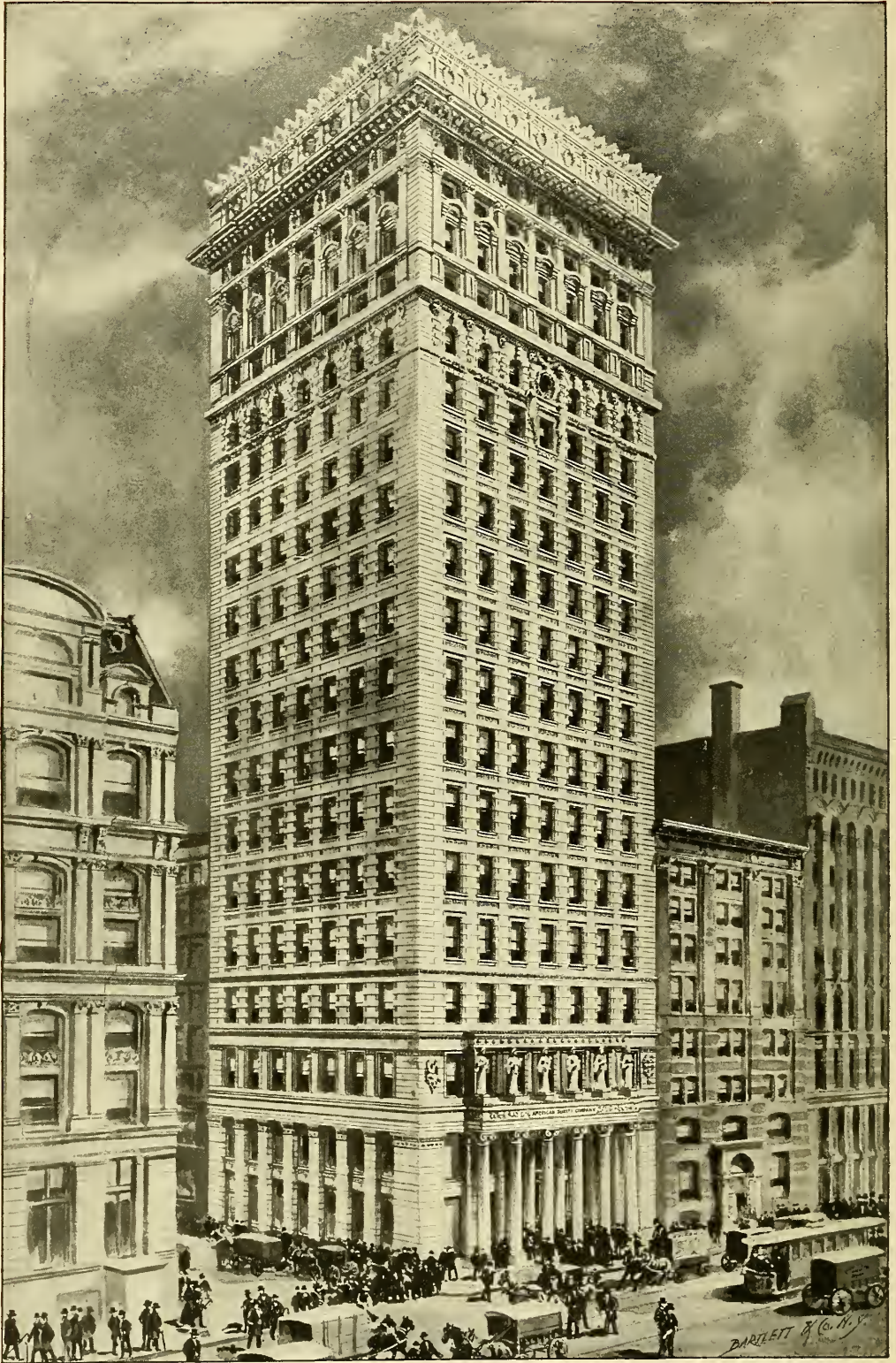
American Surety Building. 480 H.P. Babcock & Wilcox Boilers.
